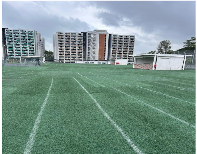
Replacing and repairing Astroturf for residents' sports activities
