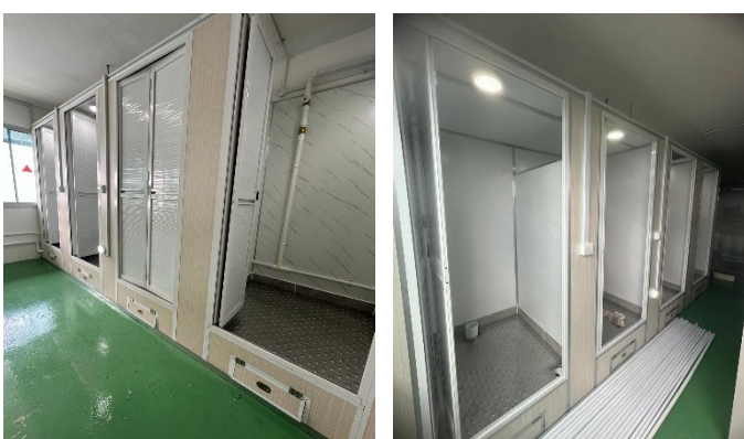
(A&A) Addition and Alteration works started at BLK 502 and 504
